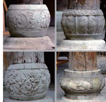
The pedestals of columns
