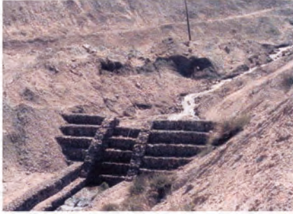
FIG. 24. Check-dam Built with Gabions
