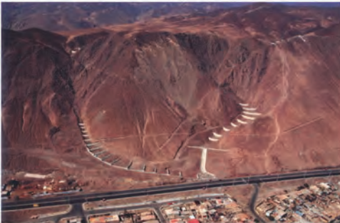
FIG. 26. Panoramic View of Chek-dams Built in Ravines El Ancla and Baquedano, Antofagasta (MOP, 2009)
