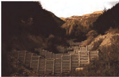
FIG. 25. Check-dams Constructed with Pre-fabricated Concrete Joists
