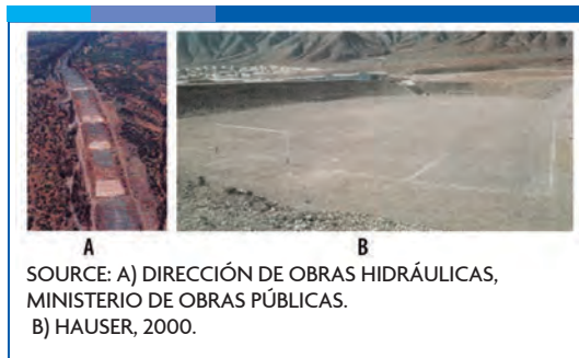
FIG. 27. Sedimentary basins. A) Aerial view of the sedimentary basins in Quebrada Macul, Santiago. B) Basin of sedimentation transformed by the community in soccer field.
