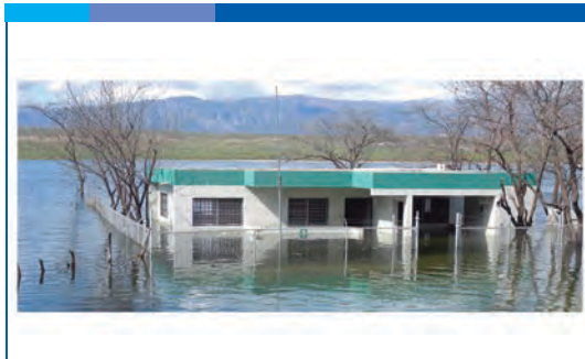
FIG. 8. Frontier Agricultural Offices Flooded by the Rising Waters of Lake Sumatra, to the West of Jimaní
