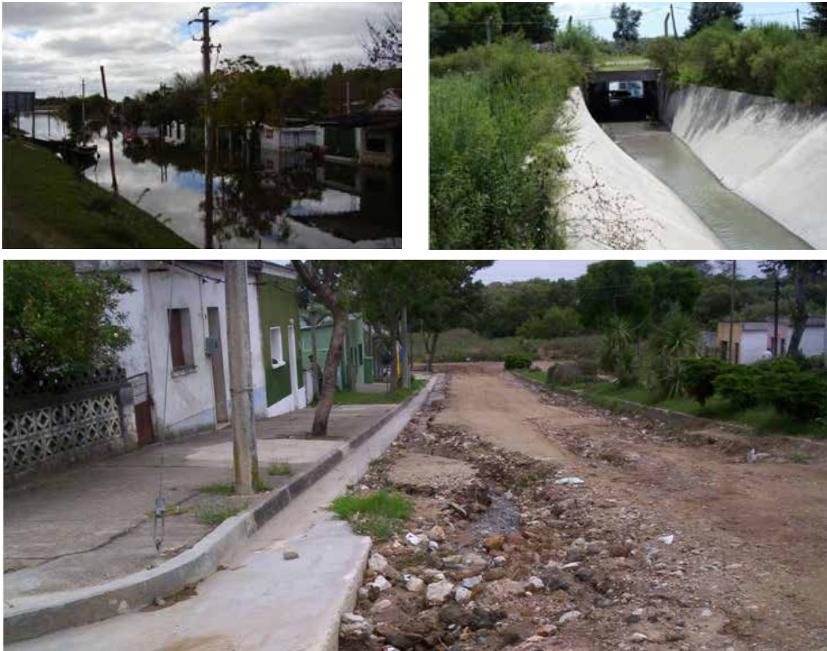
Figure 5. Rainwater drainage problems in various cities in the country
