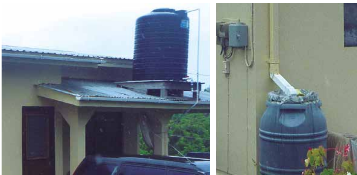
Figure 12. a) Left: Example of an elevated 500 gallon (1,890 L) black polyethylene storage tank plumbed into the home b) Right: Example of a rain barrel not plumbed into the home (Photos courtesy of Brian Neff, 2014)
