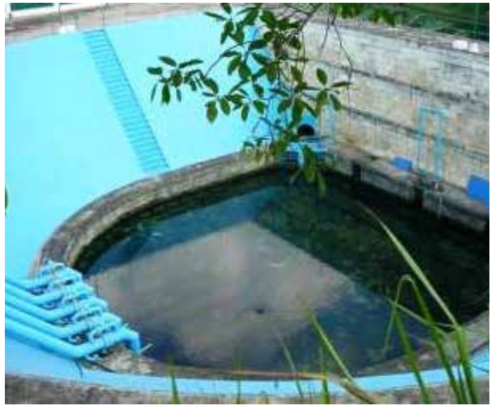
Figure 9. Vento Springs water intake today
