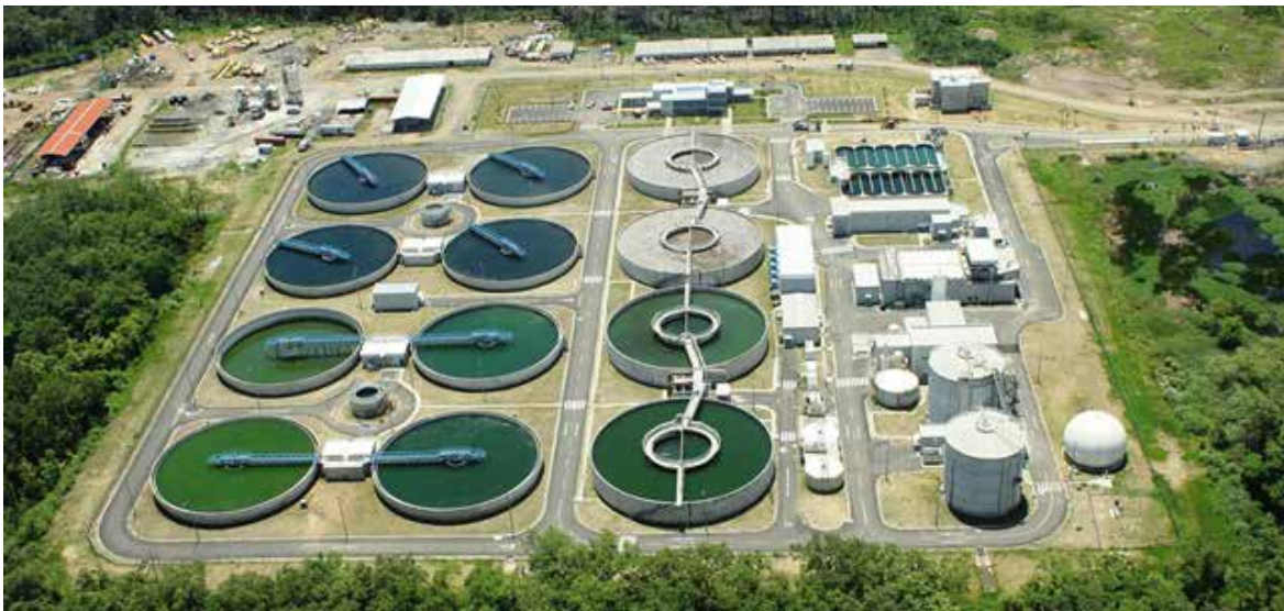
Figure 5. Wastewater Treatment Plant in Panama Bay Sanitation Project
